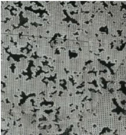
Perforated aluminium used to add depth to the facade
